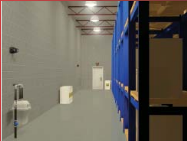
3D image showing installation of two V Series battery units and a combo unit in an industrial application under normal lighting conditions.
